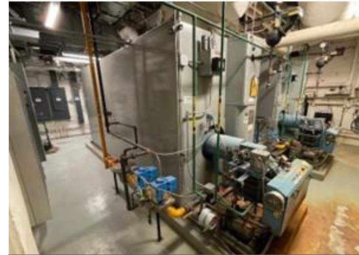
Hot Water Boilers (BOILER-1402 AND BOILER-1403)
