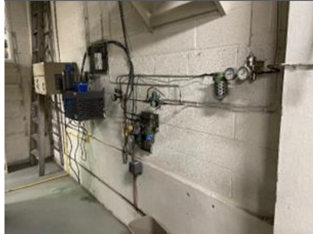
Air Dryer and Air Compressor (AIRCOMP-1401 and AIRCOMP-1402)
