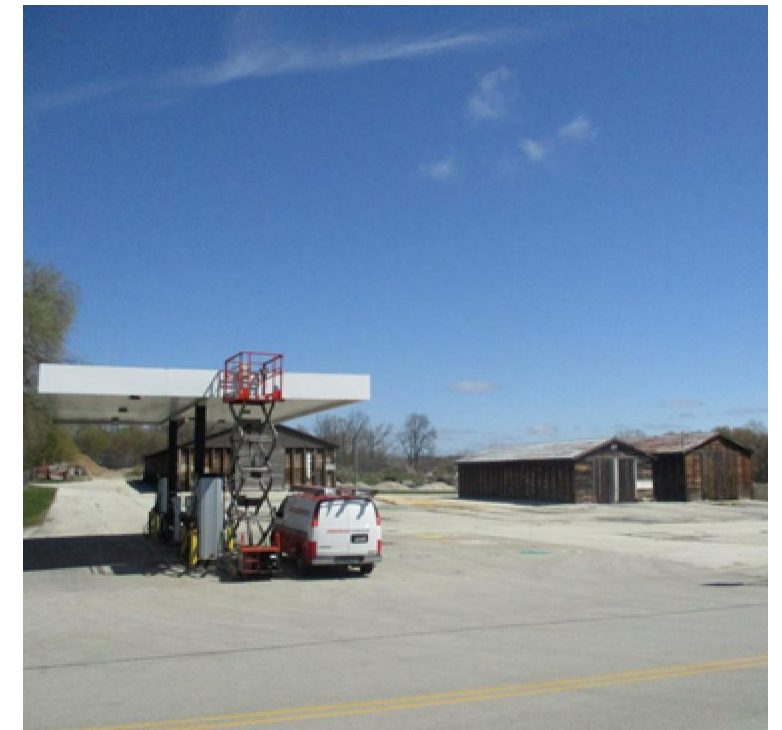
5) Pump Station /Storage Buildings
