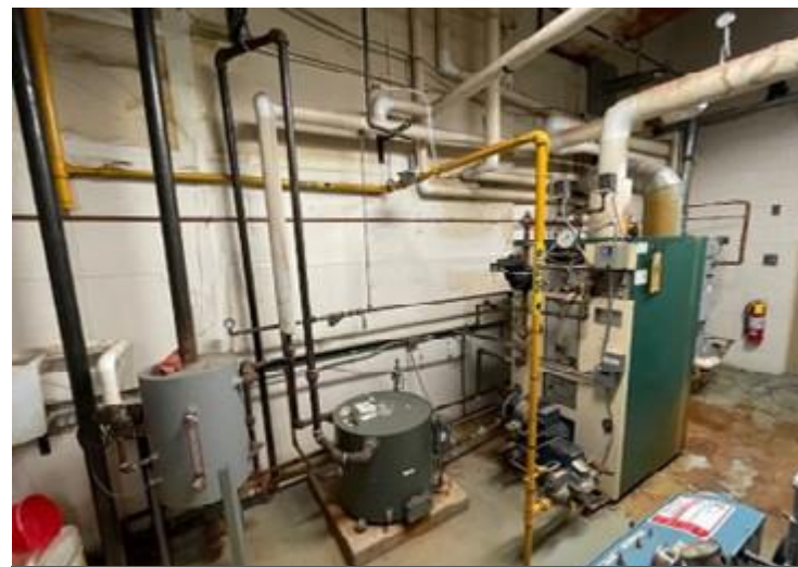
Steam Boiler for Humidification System (BOILER-1404)
