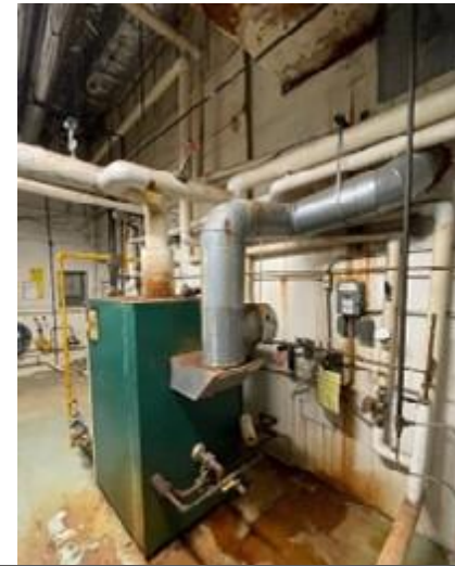
Steam Boiler for Humidification System (BOILER-1404)
