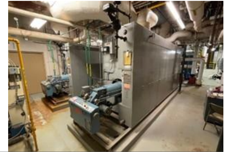
Hot Water Boilers (BOILER-1402 AND BOILER-1403)
