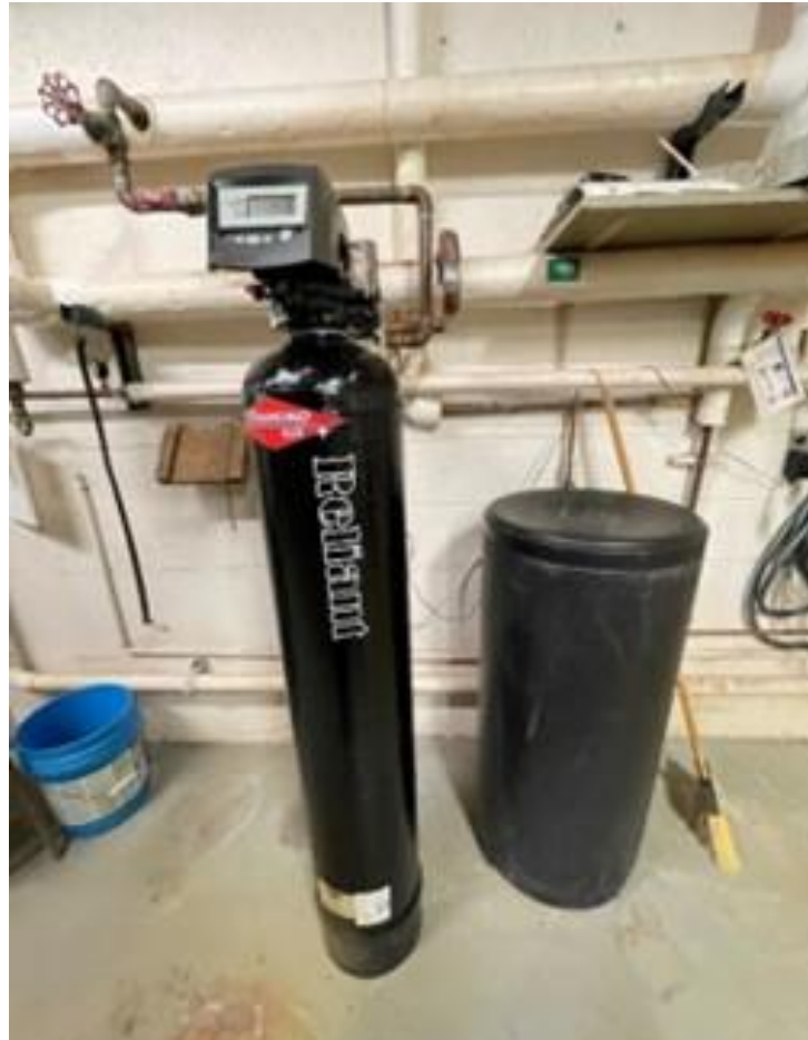
Fig. 5 Domestic Water Softener
