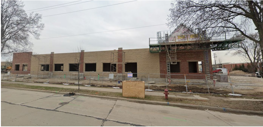
West Allis, WI (Concrete block tan and red – red is brick size)
